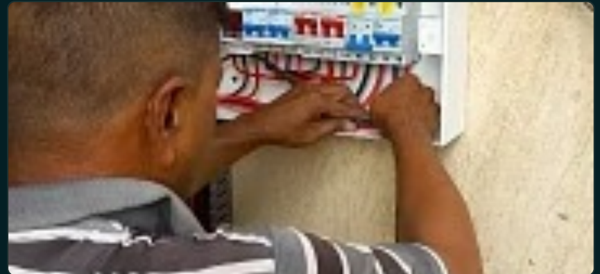
ELECTRICAL PANEL INSTALLATION — SITE WORKS
