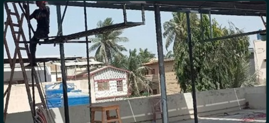
SOLAR MOUNTING STRUCTURE — SITE ERECTION
