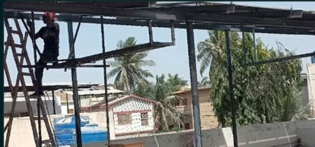
SOLAR STRUCTURE ERECTION
